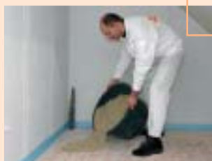
Pour onto first side of floor to be levelled
