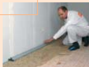
Set levelling bar on compound
