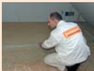
Fill between set levelling bars and tamp off
