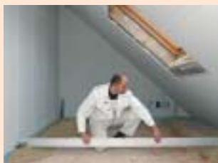
Pour out second line of compound, set second levelling bar and check level. Repeat as necessary across floor area and allow to set
