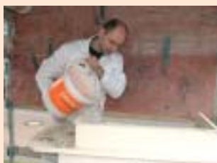
Add 12-13 litres of water per sack and mix
