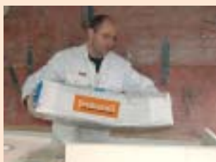
Empty sack into mixing container
