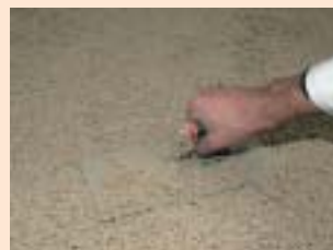
Trowel off for fine levelling
