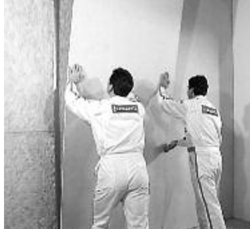
Mounting boards on a timber subframe.
