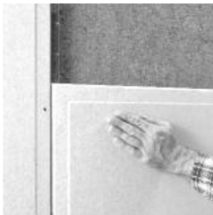
Jointing tapered edge boards.
