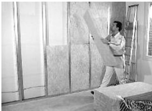
Installing mineral wool insulation batts.
