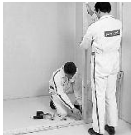
Right: Installing timber studs.
