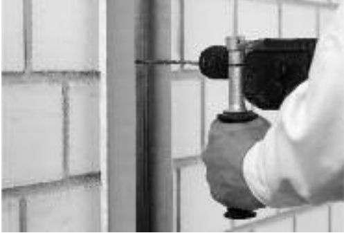
Fixing C studs to the walls with an acoustic isolation strip.
