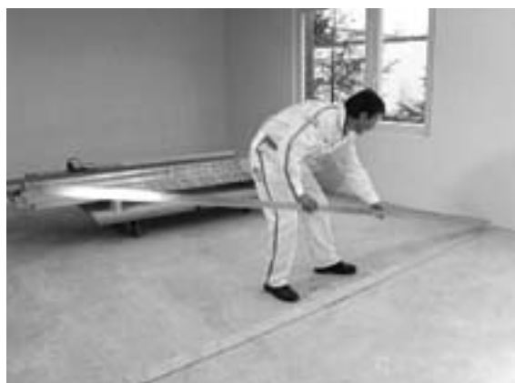
Laying the steel track sections on the floor on top of insulating strips
