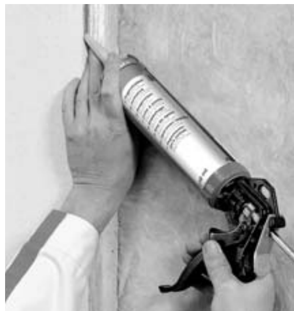
Applying the 310 ml cartridge to the board edge
