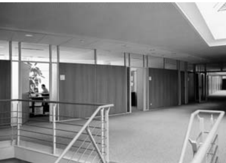
Corridor wall TFB boards veneered with real wood
