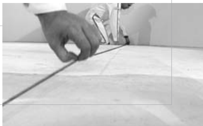
Siting the wall axes with a chalk line or construction laser
