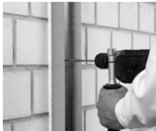
Fixing the stud on to the wall on insulating strips
