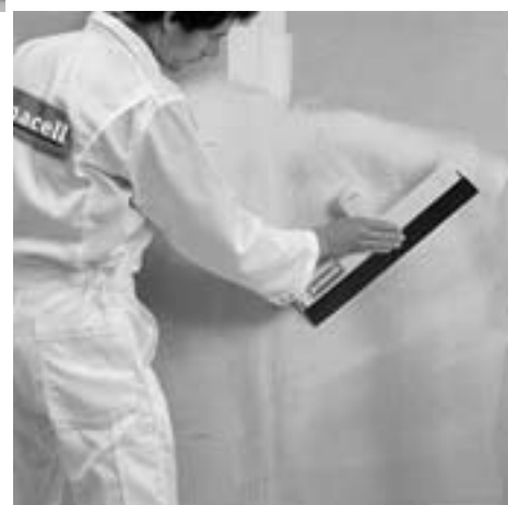
Surface finishing with FERMACELL FST
