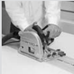
Sawing with a circular saw (with a vacuum attachment)
