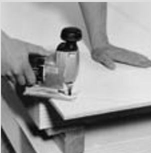
Sawing with electric jig saw
