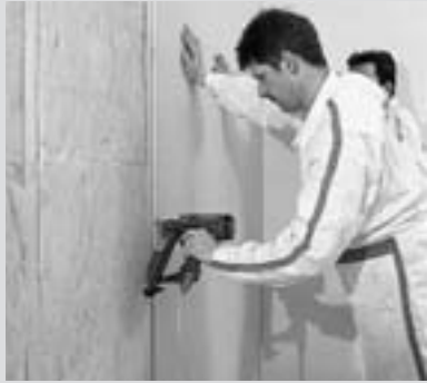
Boarding on timber studs using staples
