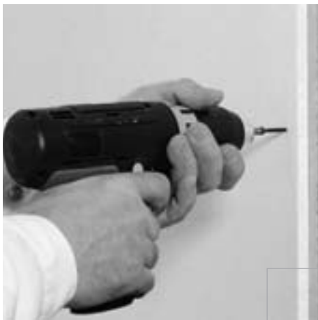
Screwing to a steel stud
