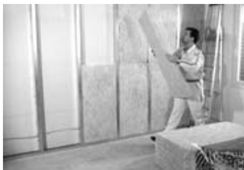
Installation of insulating material
