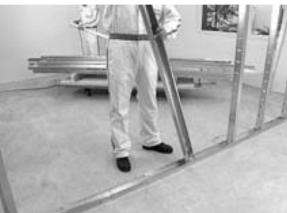
Installing the Studs
