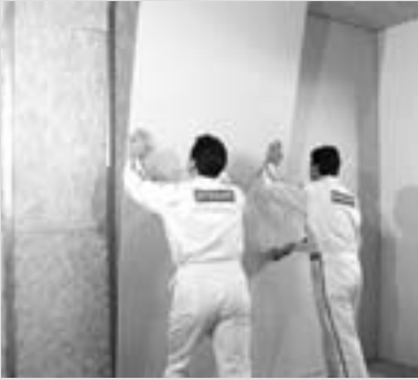
Boarding on steel studs
