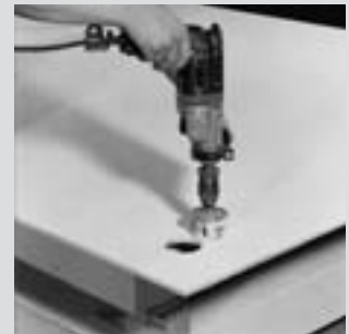
Cutting circular holes
