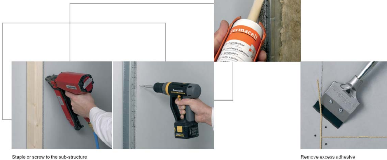
Staple or screw to the sub-structure
