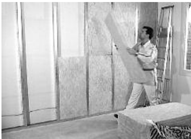
Installing mineral wool insulation batts.
