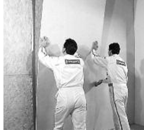
Mounting boards on a timber subframe.
