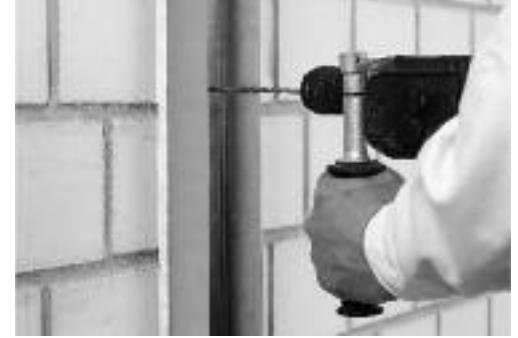
Fixing C studs to the walls with an acoustic isolation strip.
