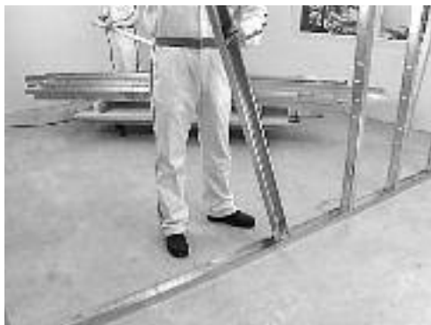
Fitting steel studs into a steel floor track.
