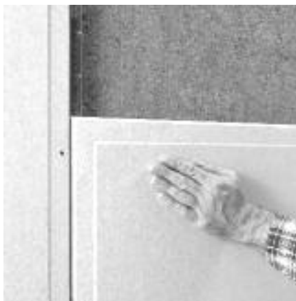
Jointing tapered edge boards.
