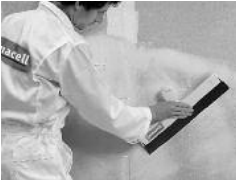
Fine surface treatment (where a smooth finish is required).
