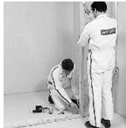
Right: Installing timber studs.
